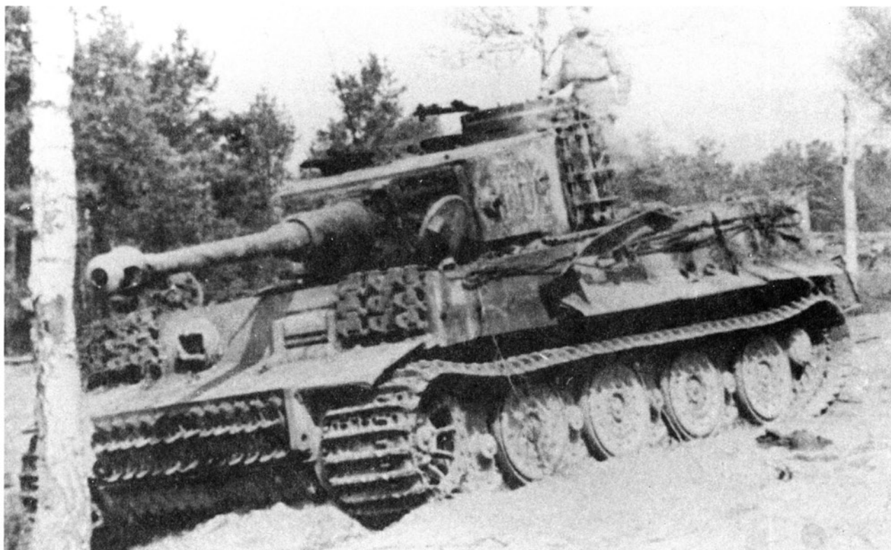
Several days later, the tank was towed to the road and recovered. The vehicle reveals a strange mixture of components, e.g., an old turret with the drum-shaped commander's cupola and the late-version steel-rimmed road-wheel suspension. BOVINGTON TANK MUSEUM
